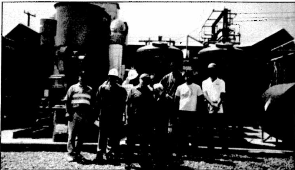
RAB members observe SFPP remediation equipment at the southern portion of Tank Farm
